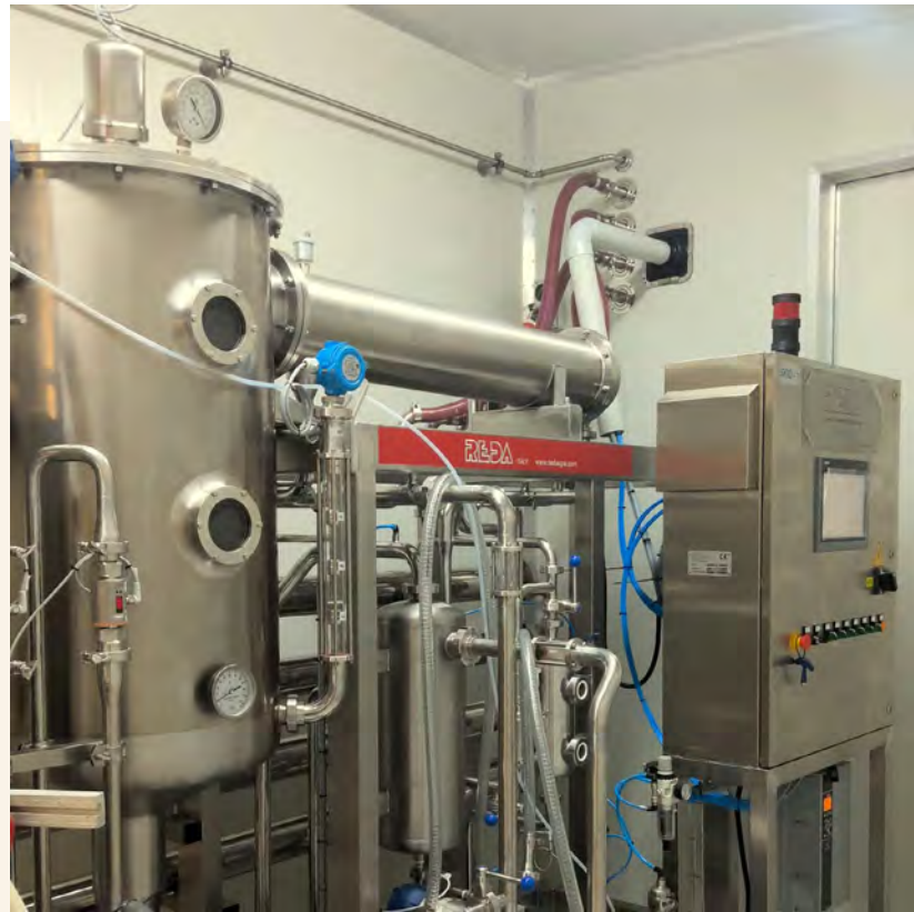
FoodSouth's new REDA low temperature evaporator
